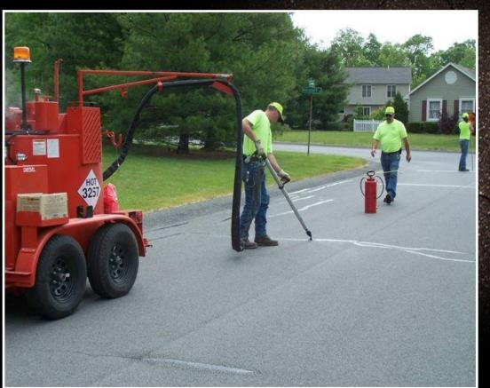
Standard crack repair treatments are an important part of all preparations work and should never be over looked.
